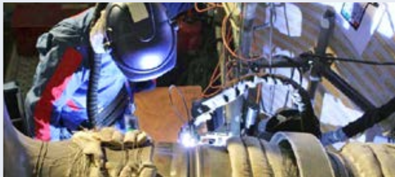
Implementation of the orbital TIG process – weld on the main secondary system
