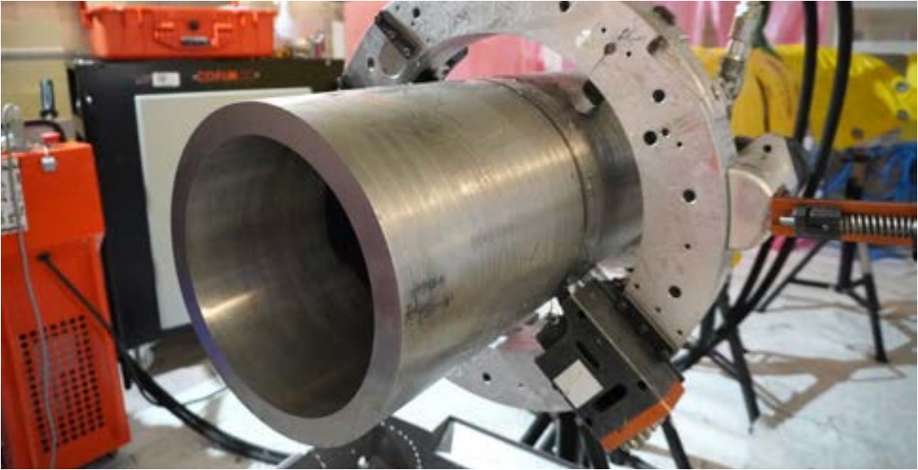
Preparation of the line before installation on the auxiliary system
